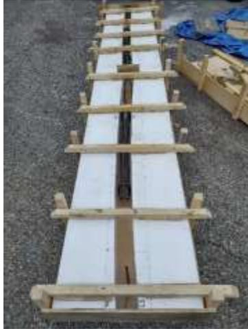
**Fig. 4** Forms for curved UHPC beams
